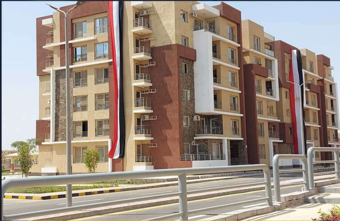
15MAY CITY "DAR MISR" (14MVA) (Residential Project)
