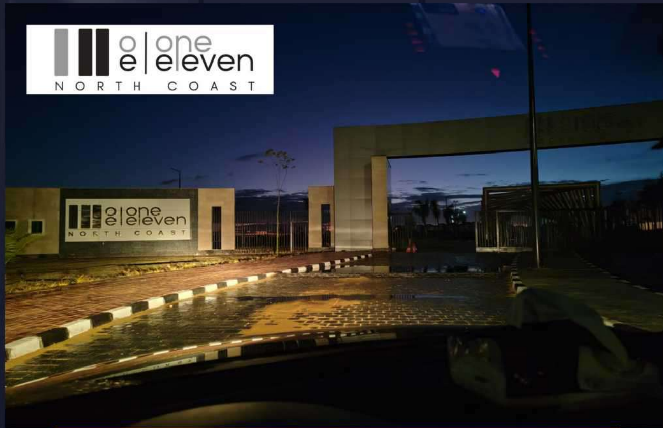
ONE ELEVEN NORTH COAST (5MVA) (Residential Project)
