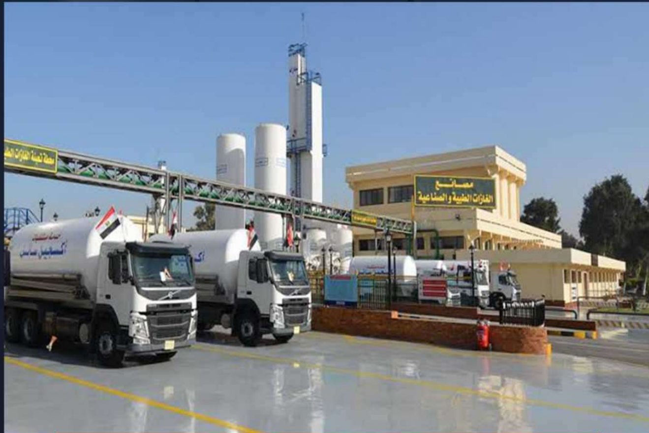
MHB INDUSTRIAL AND MEDICAL GASES (Industrial project)
